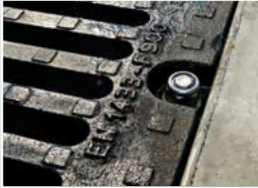
LOCKING SCREWS AND NUTS made of stainless steel
