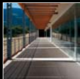
ELECTRO-FORGEWELDED GRATING
